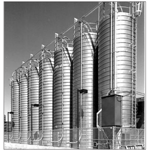
NO GRAIN IN THESE SILOS Collins built silos at the Gillette plant that hold pelletized plastic for razors and other products.
