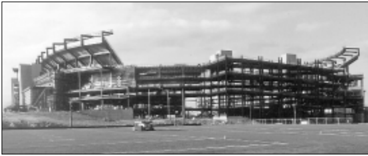
TAKING SHAPE The new CMGI Field as it was being built
