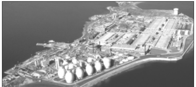
DEER ISLAND'S signature "eggs," which serve as the treatment plant's digesters, are featured in this aerial view.
