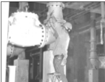
A PLUMBER tightens a bolt at the Deer Island project.
